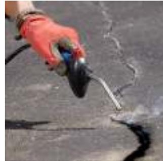
**Gambar 7. Proses *Patching or Sealing***
